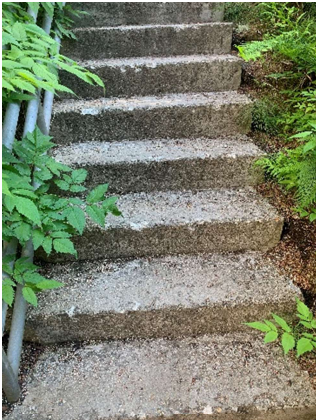
South end exterior stairs
