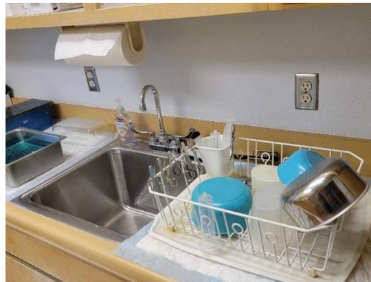
Outlets near sink
