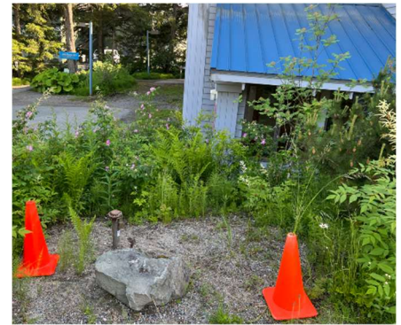
Underground storage tank location
