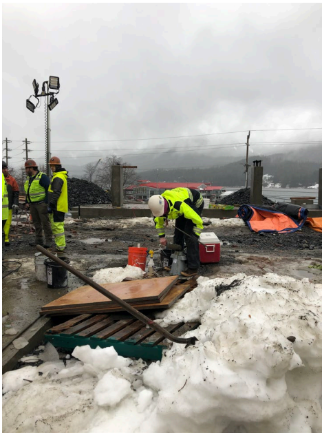
10. Placement continuing along GL AA. Vibrators at GL4.
