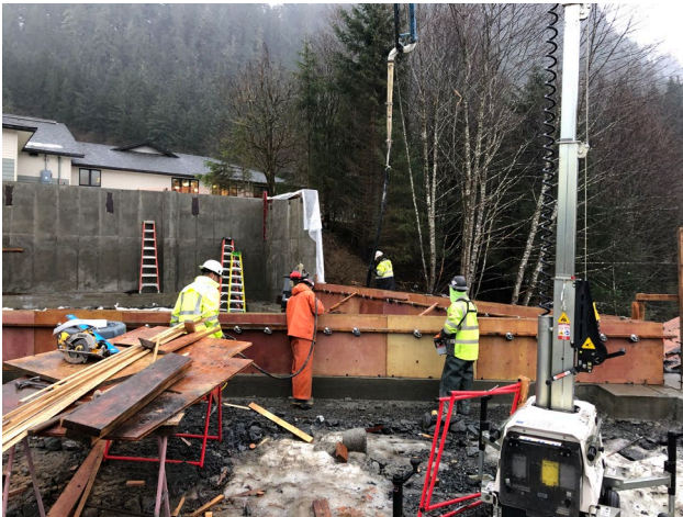
12. Second lift in progress at GL AA, followed by vibrators.
