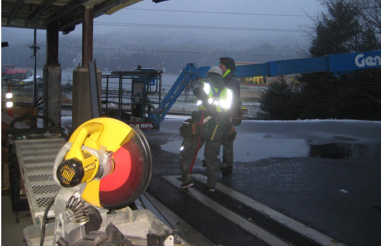
Photo 2845 – DC workers, Trevor and Spencer, cut and load fiberglass girts onto to the lift in advance of installing them to the building's west façade.
