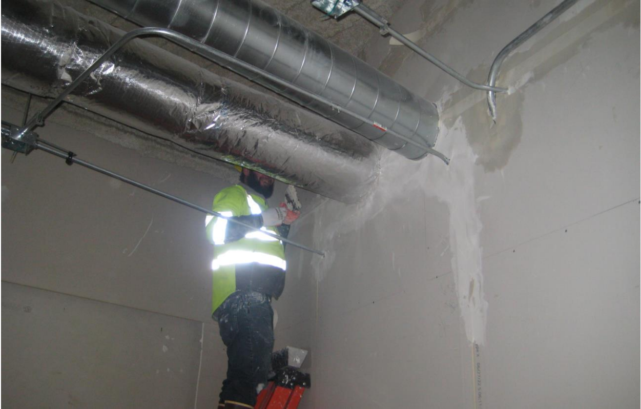
Photo 2849 – CC drywall worker, Mike, applies tape and mud to the upper portions of the interior walls within a room on the second floor level level.
