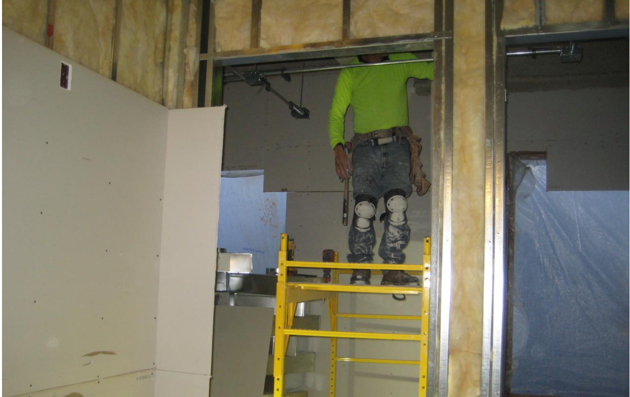
Photo 2847 – CC workers, laborers, install sheetrock to the interior walls within room 221, Provider Office, on the second floor level.
