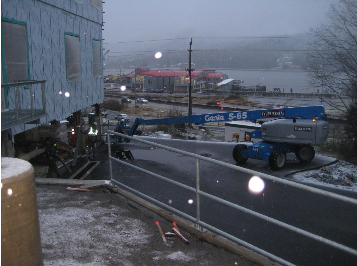
Photo 2844 – DC workers, Trevor and Spencer, utilize the 65 foot man lift in preparation to install fiberglass girts to the building's west. White 'dots' are snowflakes.
