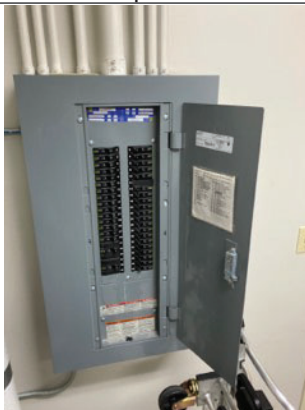
Main 800 amp electrical service panel with sub panel disconnects
