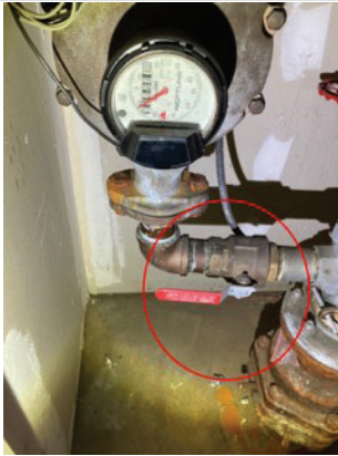
The main water shutoff valve is located in then sprinkler riser closet in the front , street side corner of building accessible through BRH space.
