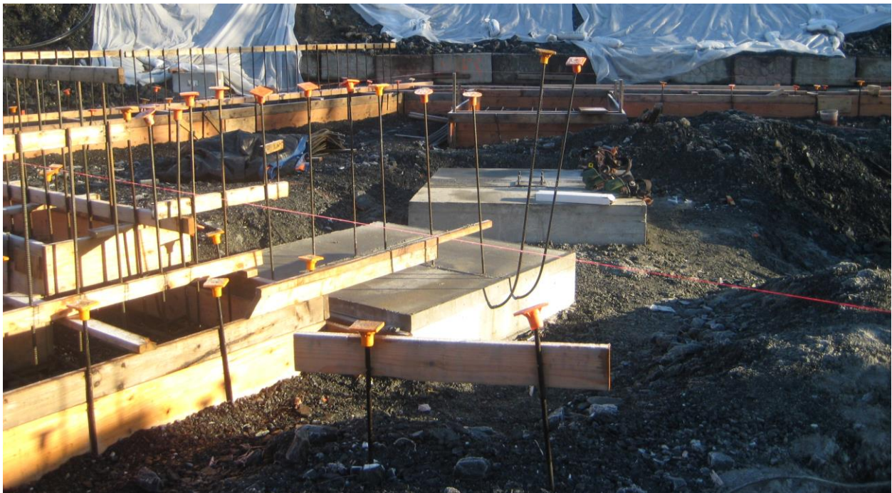
Photo 0963 – Partial overview of site showing completed concrete placement along GL E and EE.
