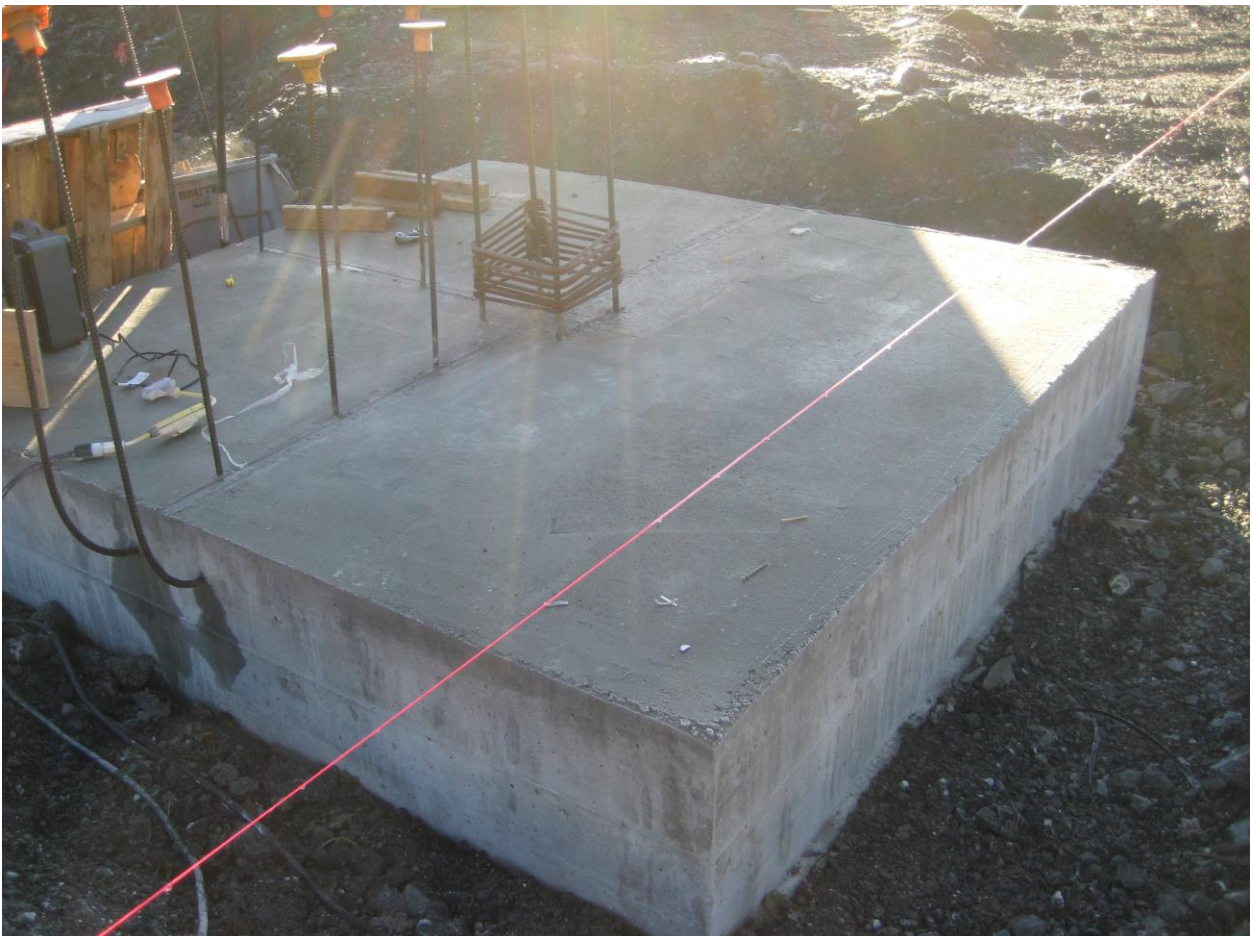
Photo 0965 – Photo of spread footing at the intersection of GL's D and 3.
