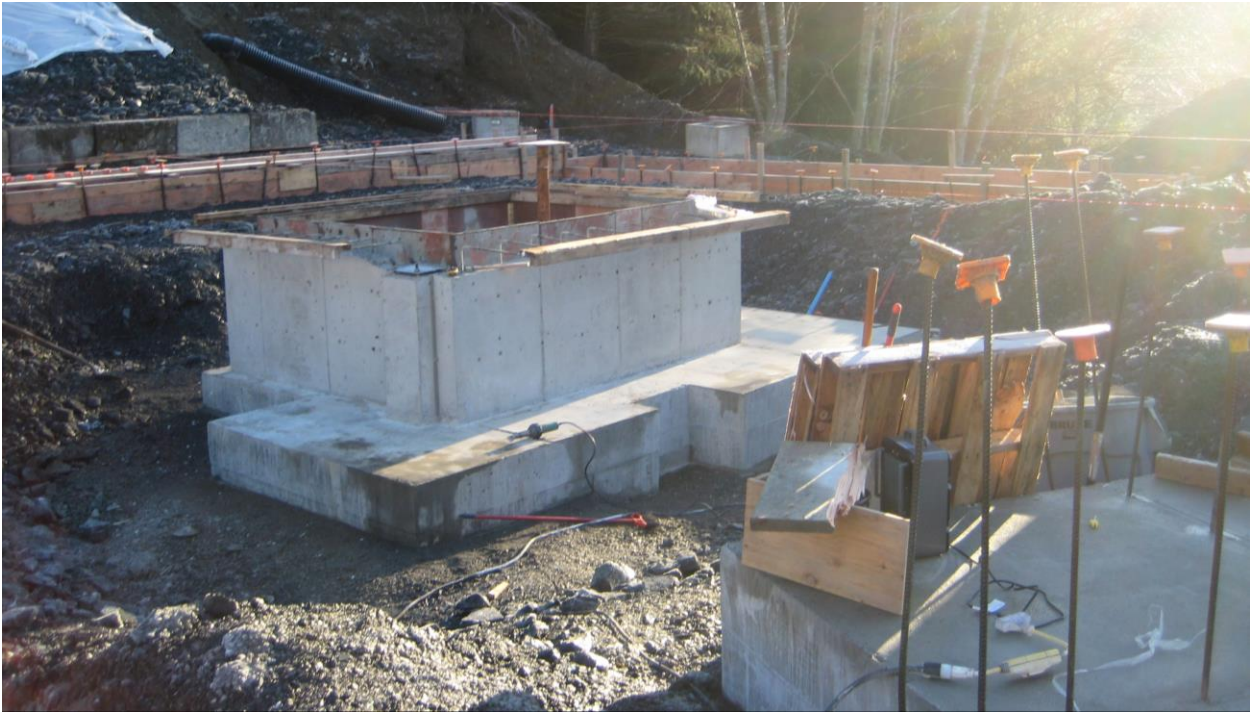
Photo 0964 – Photo of elevator pit walls prior to covering with waterproofing materials.
