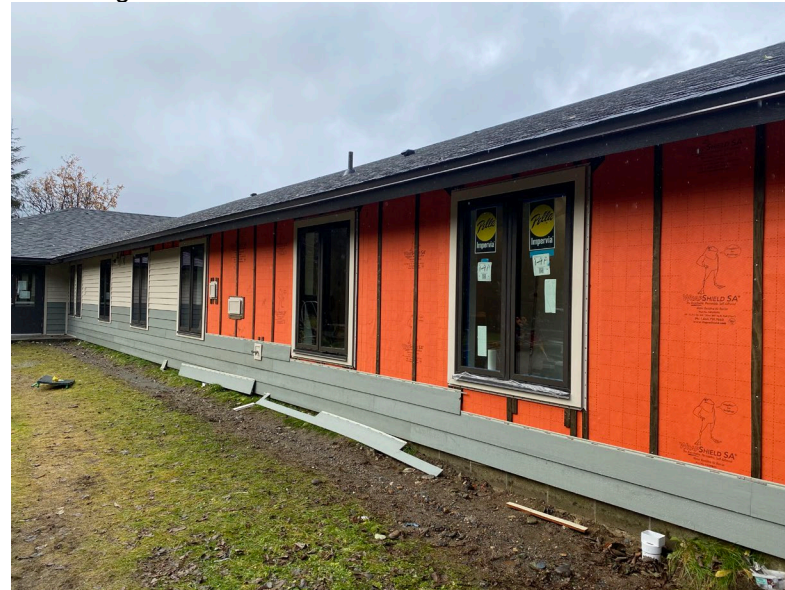
2. Siding extent at south elevation
