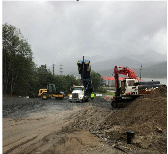
3. Line of excavation at SW portion of building near existing 12" DI water line.
