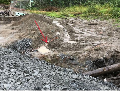
4. Ponding at bottom of excavation due to heavy rain.
