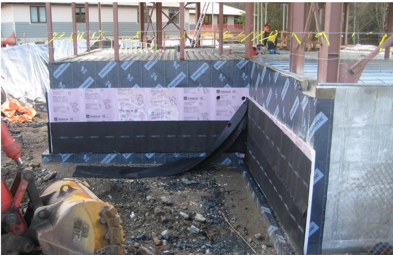
Photo 1684 – As noted in yesterday’s report, the geo-tech filter fabric along the exterior face of wall on GL “2” has failed. Will require repairs prior to backfilling.
