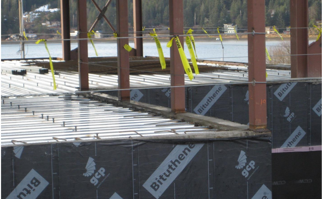
Photo 1680 – Another view of edge condition with wall and rebar (tie) interface.
