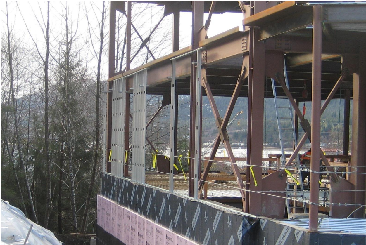
Photo 1685 – DC workers (Alex and Riley) have started a portion of the exterior (metal stud) wall framing along GL “8”.
