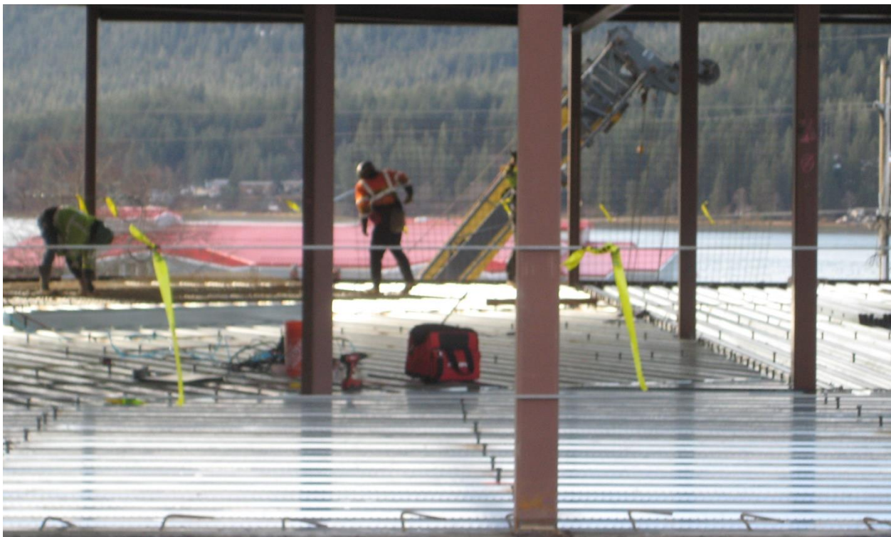
Photo 1682 – View of edge condition at GL “F”. Note that CC workers have installed (epoxied) rebar into the upper portion of the basement wall to provide a ‘tie’ between the wall and slab.
