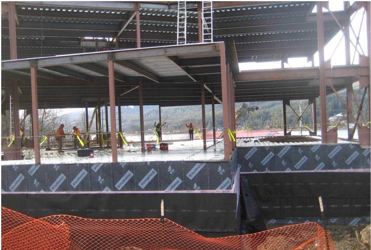
Photo 1679 – Group photo of all three-subcontract firm's (DC, CC and IP) work crews on level one pan deck. Note that CC workers are placing and tying reinforcement mat in background.
