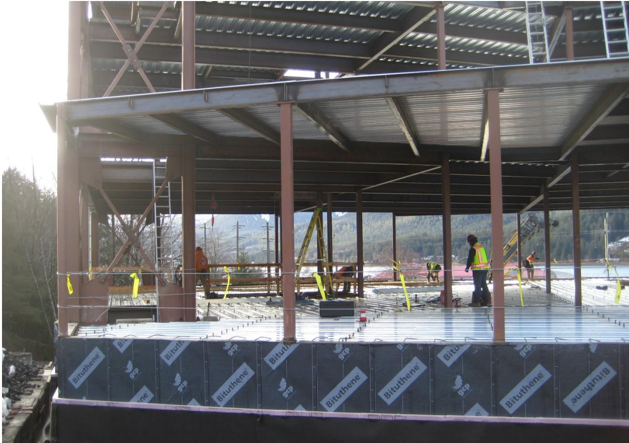
Photo 1683 – IP worker (Kyle) performs ‘mechanical/plumbing’ layout on level 1 pan deck (in foreground.) Two CC workers place and tie 4 x 4 WWM reinforcement in background.
