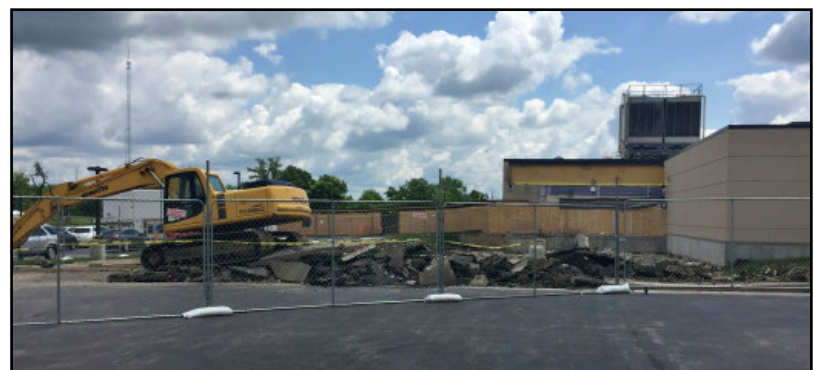
The $2.3 million expansion will provide 7,000 additional square-feet within Medical Imaging and shell space for future Emergency Department expansion.
