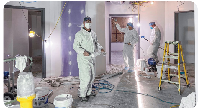
Our skilled POM staff continue construction for the new Behavioral Health Unit, set to open spring 2021.
