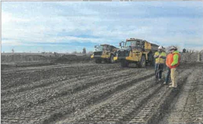
*GeoProfessional Innovation on site inspecting the placement and conditions of the structural fill for the building pad.*
