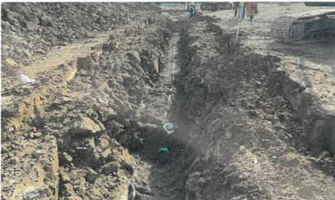
*Big D's installing the sanitary sewer line.*
