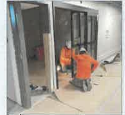
Perfection installs sliding doors
