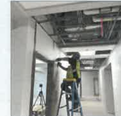
PCI installs wall panels
