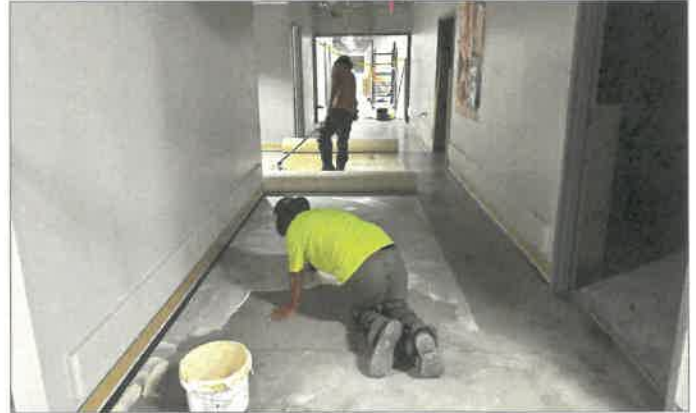
Great Floors installing vinyl sheets in Area B.2 Corridor.
