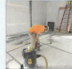
Brayden installs MRI anchors
