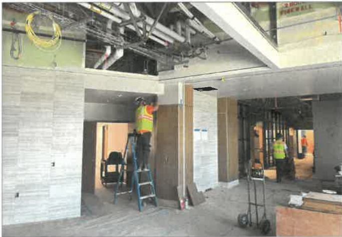
PCI installing wood paneling at Area C Public Corridor.
