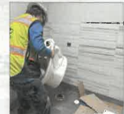
AMC installs plumbing fixtures
