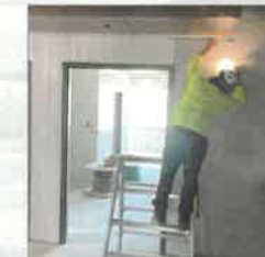
Paintmaster installs wall paper
