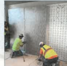
GEC installs light box
