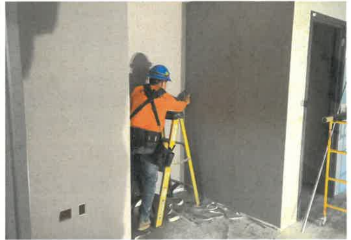
Paintmasters installing wallcovering at Area E Alcoves.
