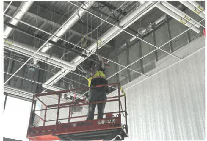
Garrett Electric roughing-in lights are Area C Lobby.
