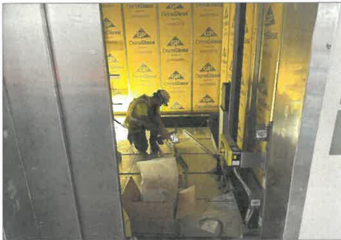
Otis continues to install public elevators in Area E.
