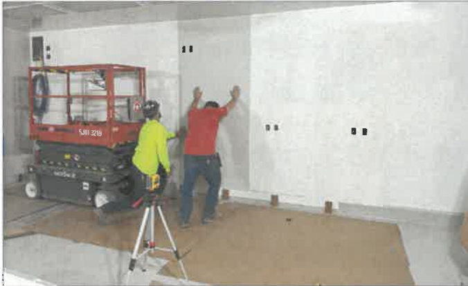
Bouten installing wall protection in Area B.2 OR 1.
