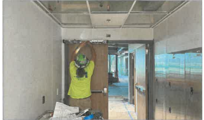
Division 8 installing door operators in Area C kitchen.
