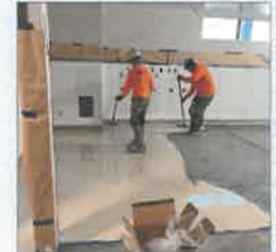
Paintmaster installs epoxy floor
