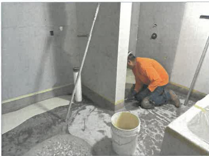
Columbia Industrial Coating installing epoxy in LDRP Bathroom in Area F.
