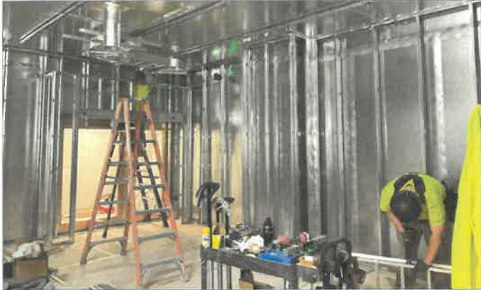
Garrett Electric installing cable tray at Area B.1 MRI Room.
