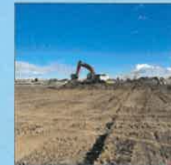
Clearing and grubbing site
