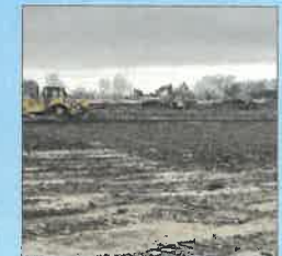
Starting building pad
