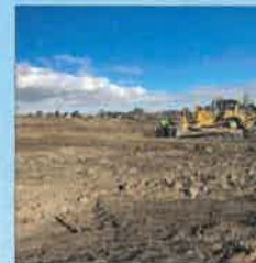
Starting building pad
