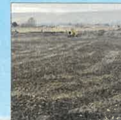
Proof rolling building pad
