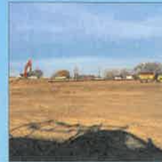
Clearing and grubbing site
