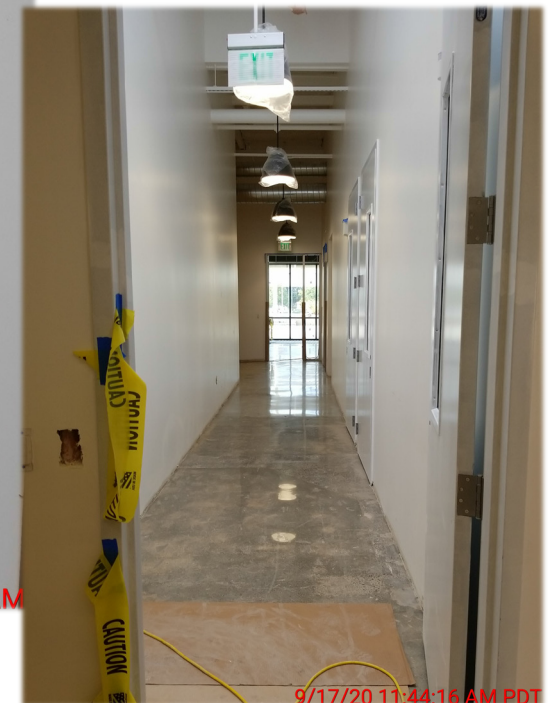
Hallway (looking toward front door)
