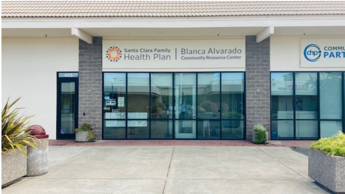
Front of Building
