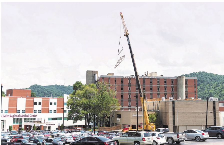
A new roof structure for the former Morehead Clinic building is taking shape as St. Claire Regional prepares to renovate the entire structure. Next will be the staining of the white exterior brick on the smaller building to match the hospital's exterior coloring. (Caption and photo by Cory Claxon, The Morehead News)
