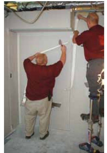
Facilities management staff members, Larry Hamm (left) and Jeremy McCleese (right) finish drywall in the Women's Imaging Center.
