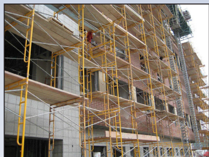
Masonry work on the exterior of the building nears completion
