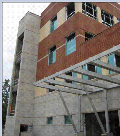
Windows and exterior structural steel are being placed.
