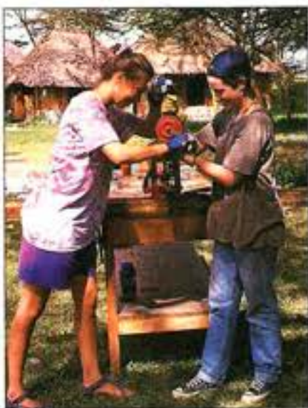
Practical problem-solving is put to a test as students design and construct a bird observation tower for use in their directed research project. Student bandas (living quarters) can be seen in the background.
