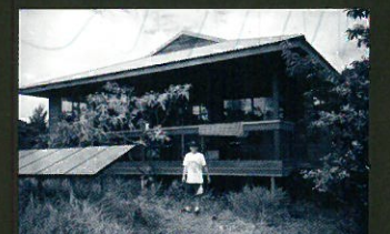
Structures and Solar Equipment
