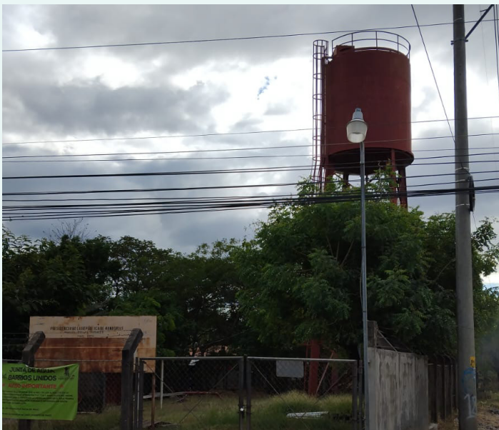
This water storage tank is contaminated and unreliable, as it cannot provide enough water for everyone throughout the year.
