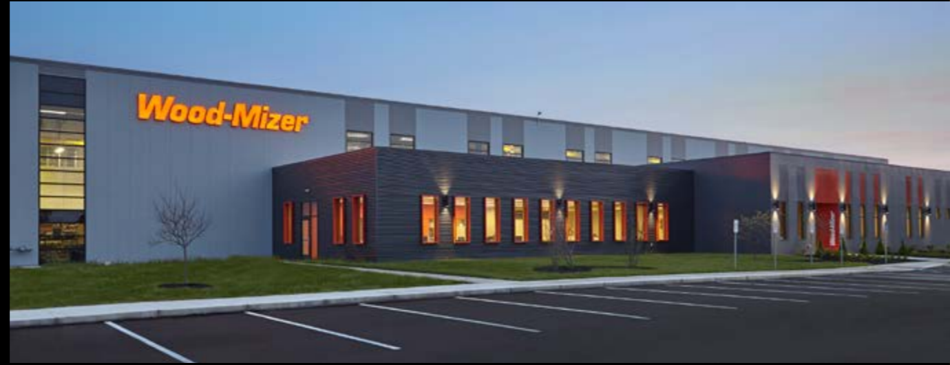
Wood-Mizer US Headquarter's new production hall in Indiana.
