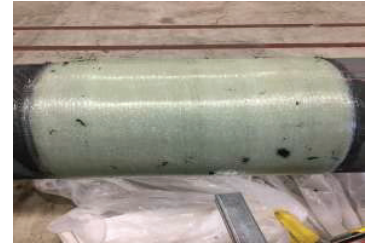
View of Repair
