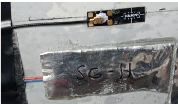
Figure 3: Dragonfly sensor before protective layer installation
