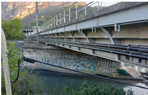
Figure 1: The railroad bridge monitored. The external metal girder on which the sensors are installed is visible.
