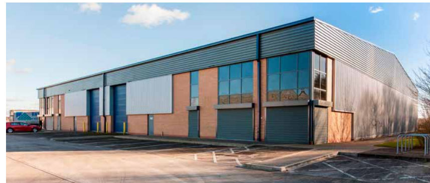
New DPD Distribution Hub completing Spring 2018
