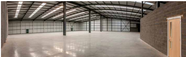
New DPD Distribution Hub completing Spring 2018
