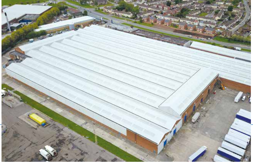
Fully Refurbished Roof with 25 year warranty
