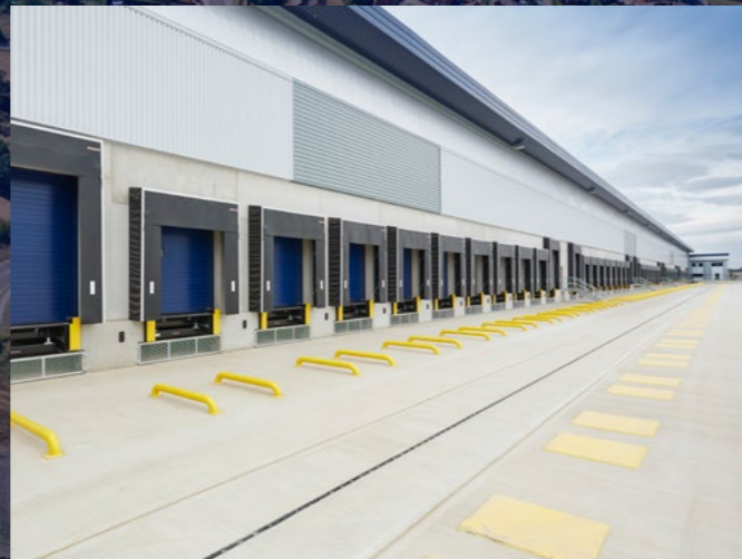
Markham Vale Exterior
