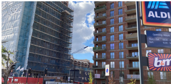
5. Partially constructed residential blocks opposite the site
