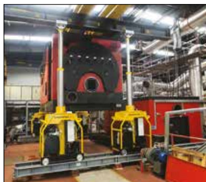
▼ Moving and positioning a 25 tons boiler using the ML40 Mini-Lift Gantry.
