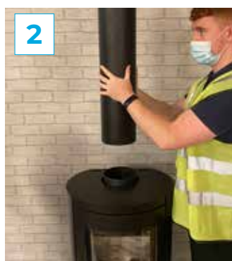
Extend pipe into the stove spigot and seal with high temp sealant
