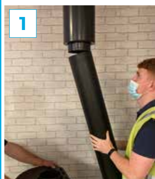
Slide pipe into TWPro connecting starter length
