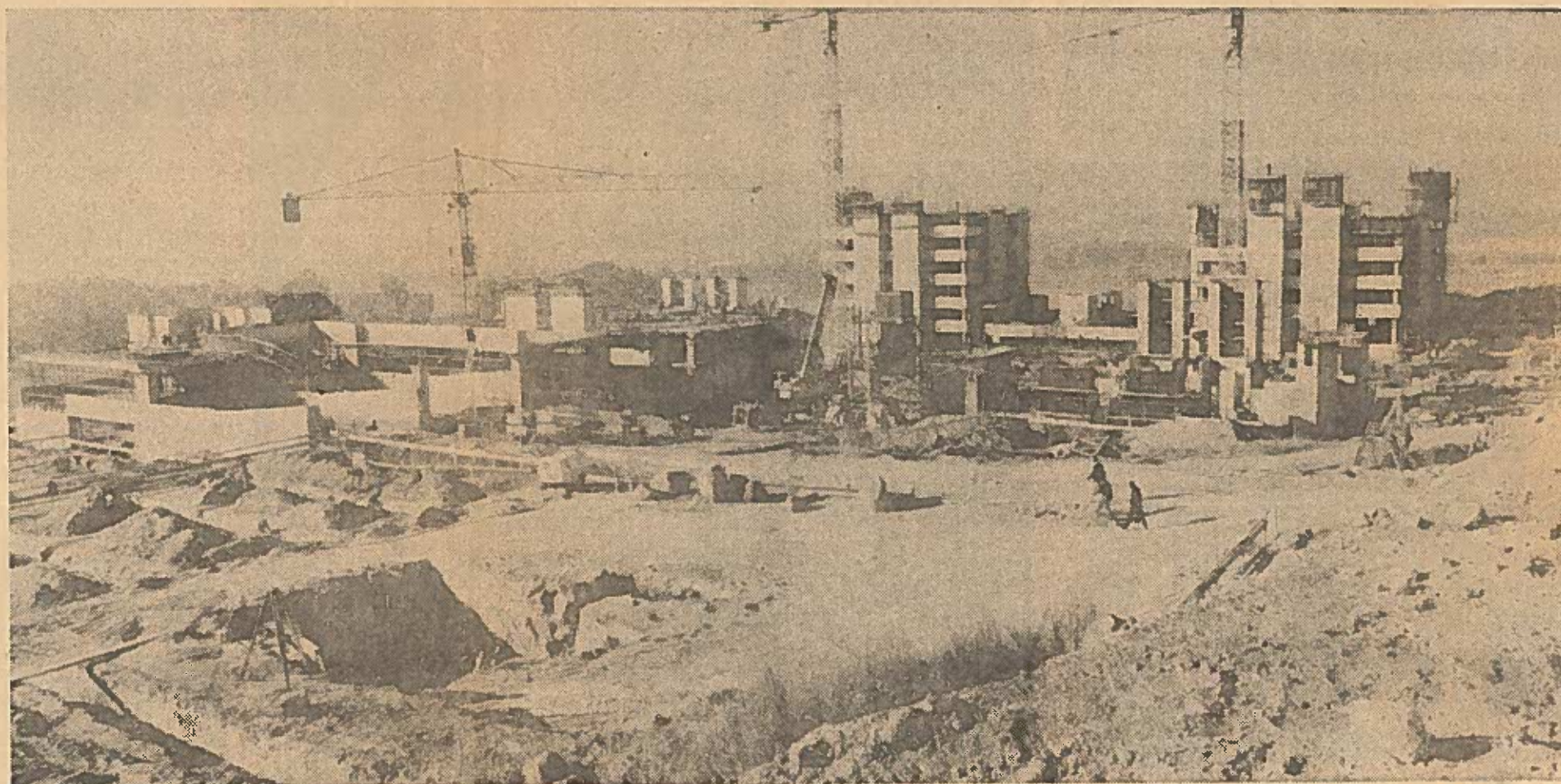
This site in western Pretoria used to resemble a vast veld wasteland. Chosen to house the new Pretoria Technikon, it will eventually be turned into a natural paradise interspersed with large modern concrete structures. Under construction are two women's hostels on the right. In the background, not visible, are the sports fields. The classrooms and administrative buildings will be built to the left of this photograph.
