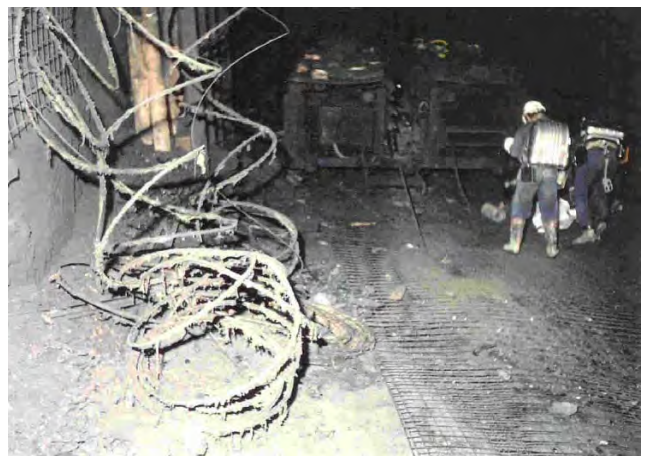
Figure 21.14C Photographs of post-explosion No.1 Surface Portal, dislodged and damaged steel arches, and remnants of ducting. Westray Mine Public Inquiry, Exhibit No. 59 (Richard, 1997).
