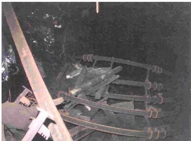
Figure 21.14C Photographs of post-explosion No.1 Surface Portal, dislodged and damaged steel arches, and remnants of ducting. Westray Mine Public Inquiry, Exhibit No. 59 (Richard, 1997).
