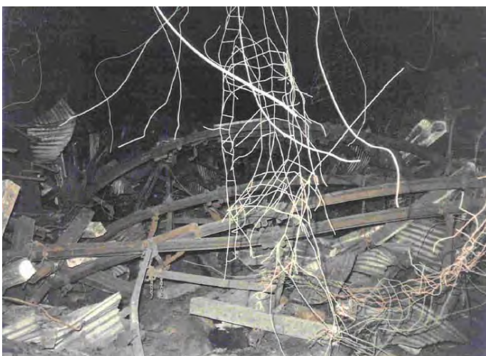
Figure 21.14D Photographs of roof falls, dislodged steel arches, and damaged equipment. Westray Mine Public Inquiry, Exhibit No. 59 (Richard, 1997).
