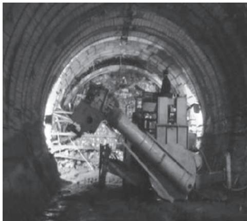
Figure 5. Casagrande PG 175 drilling rig at work.
