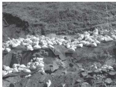
Figure 2. Arrangement of muffling for control of flyrock.
