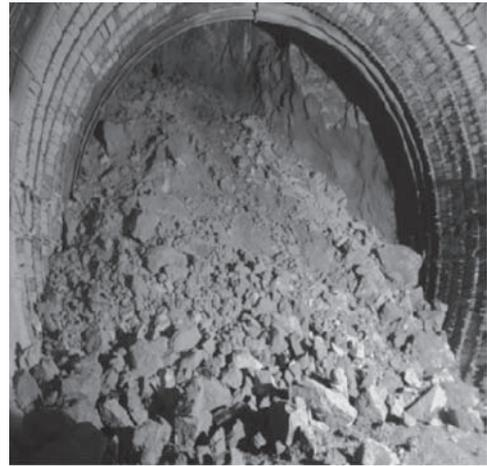
Figure 2. Loose fall from left SPL to crown.
