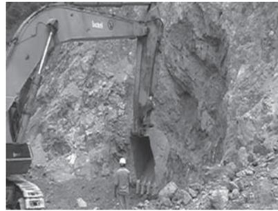
Figure 7. Tunnel portal excavation by excavator.
