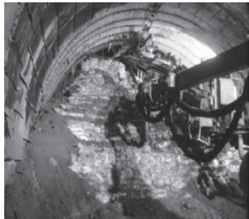
Figure 3. Forepoling with 36 mm steel rod using Boomer.
