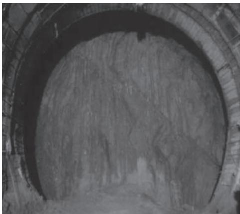
Figure 6. Full face of modified horse shoe shape.
