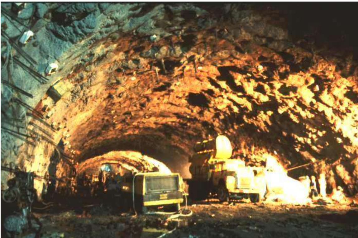
Figure 19: Completed excavation of the cavern arch.
