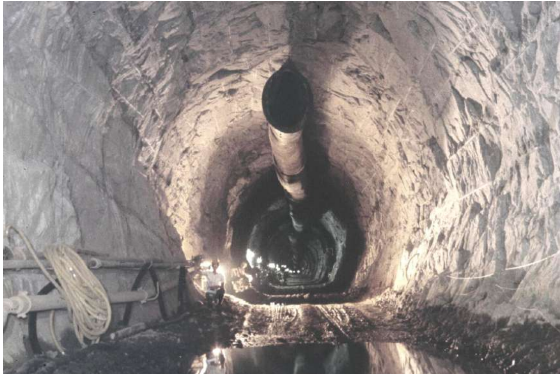
Figure 5: Results achieved using well designed and carefully controlled blasting in a 19 foot diameter tunnel in gneiss in the Victoria hydroelectric project in Sri Lanka. Note that no support is required in this tunnel as a result of the minimal damage inflicted on the rock. Photograph reproduced with permission from the British Overseas Development Administration and from Balfour Beatty - Nuttall.
