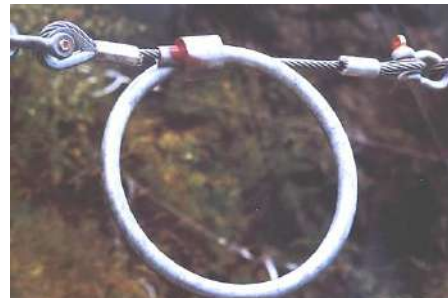
Figure 6: Details of a rockfall net system manufactured by Geobrug of Switzerland.
