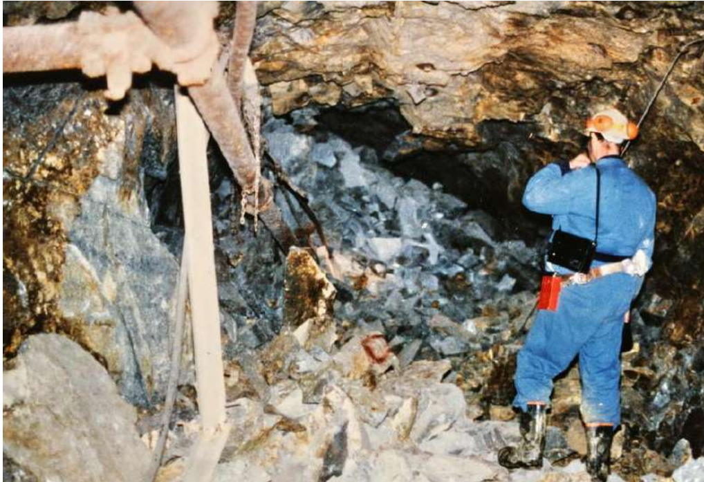
Figure 3: The results of a rockburst in an underground mine in brittle rock subjected to very high stresses.
