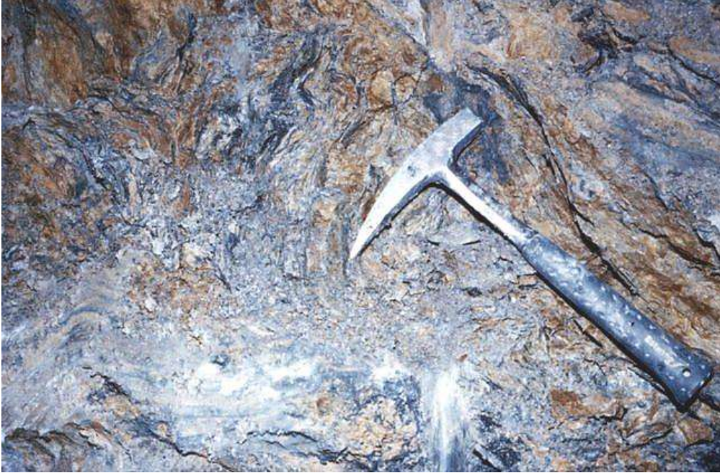
Figure 28: Appearance of the very poor quality Athenian Schist at the face of the side heading illustrated in Figure 27.
