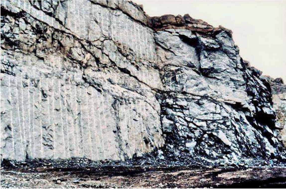
Figure 6: Comparison between the results achieved using controlled blasting (on the left) and normal bulk blasting for a surface excavation in gneiss.
