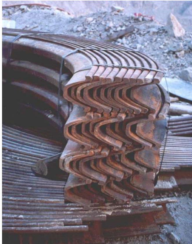
Figure 13 Top hat section steel sets delivered to site ready to be transported underground.
