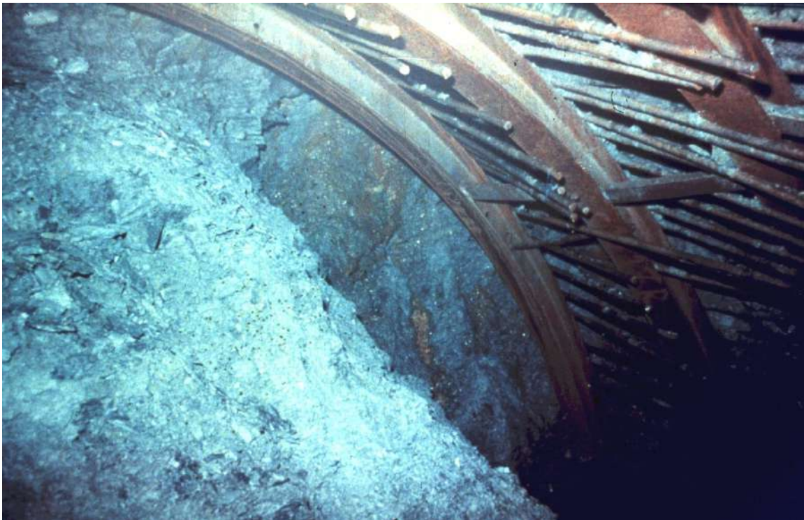
Figure 19: Spiling in very poor quality clay-rich fault zone material.
