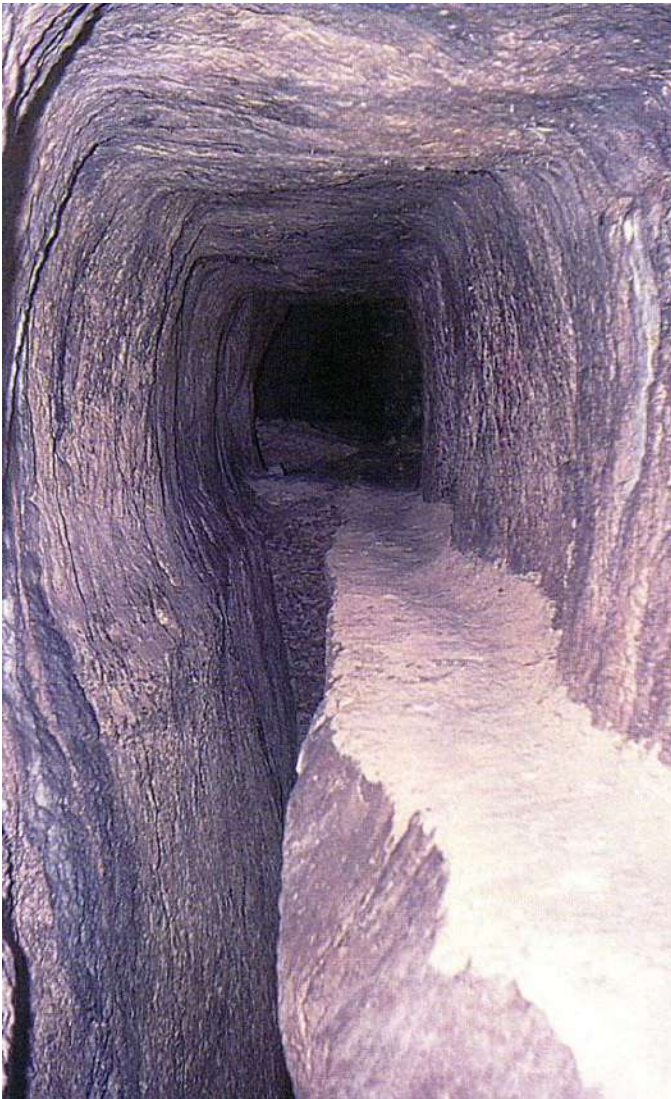
Figure 5: The 1036 m long Eupalinos water supply tunnel was built in 530 BC on the Greek island of Samos. This is the first known tunnel to have been built from two portals and the two drives met with a very small error.
