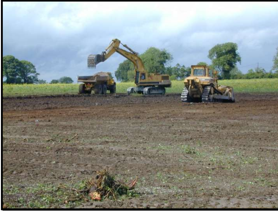
Plate 2 – Soil stripping by backhoe and dumptruck
