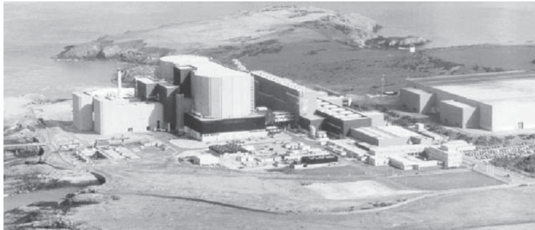
Figure 7.12 Power station project.
