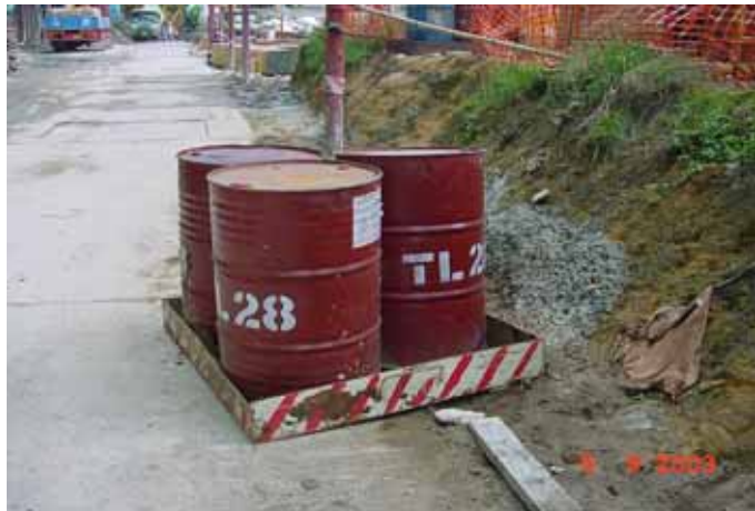
Bundled tray to prevent spillage from the container
