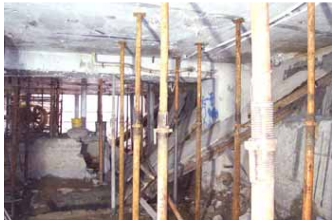
Install steel propping under slab & beam.
