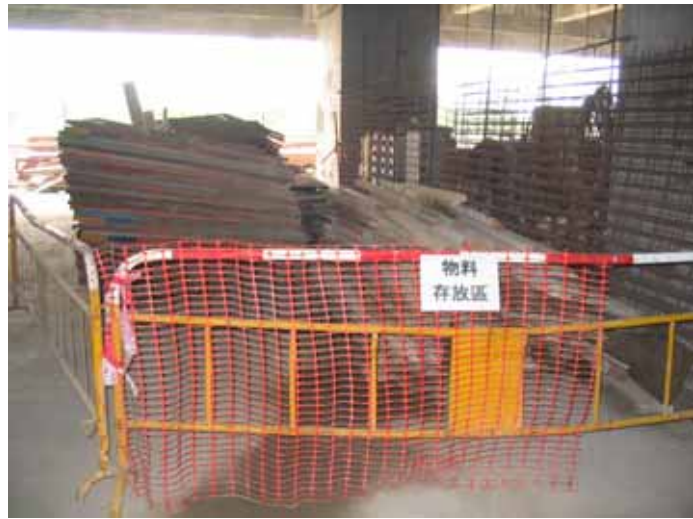
Proper stacking in a temporary storage area
