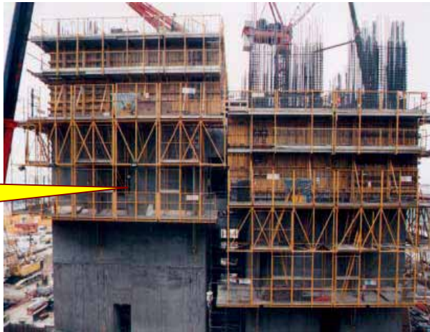
Working platforms at various decks
