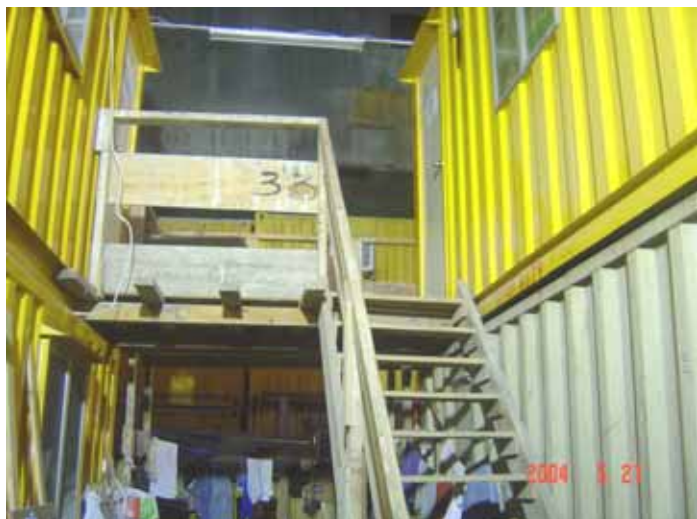
Container provided on worksite for subcontractors' work and rest
