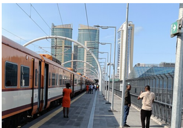
Modern railway station in Dar es Salaam city center
