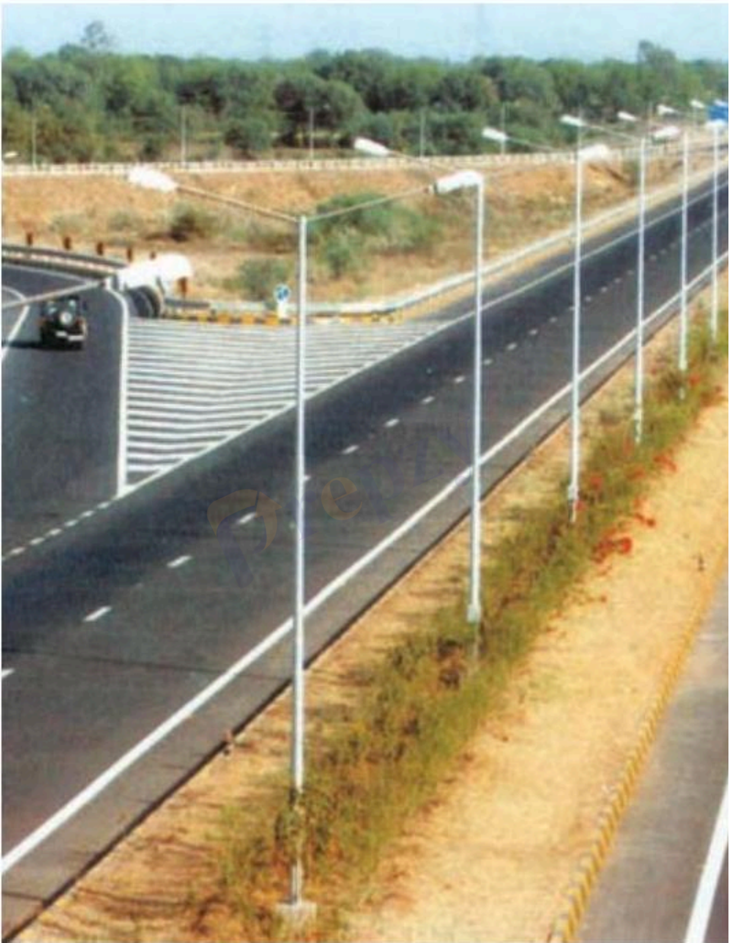
This expressway features divided carriageways separated by a median strip with greenery and streetlights, enhancing safety and visibility. T entry and exit. Such highways are designed considering speed, stopping distance, friction, and lighting to ensure safe and efficient travel.
