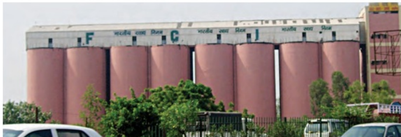
Fig. 1.10 (a) : Silos for storage of grains
