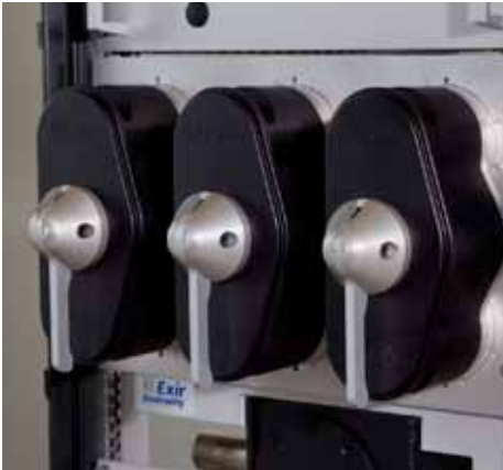
1. Example of Splitter Panel in normal mode.
