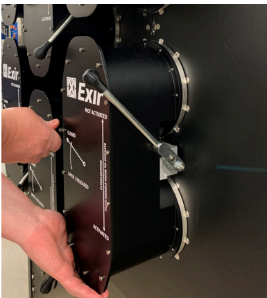
4. Continue until the right handle is in the upper position and prepare to release the left handle. The U-link is still fixed with contact pressure.
