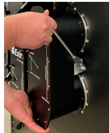
3. Continue to pull the handle upwards. This movement will affect the interlocking for a safe operation.
