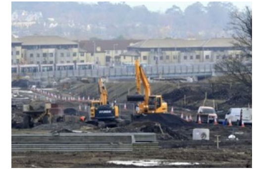
Construction is underway in Cherrywood in South Dublin of a new ‘town’ that will accommodate an estimated 25,000 people.
