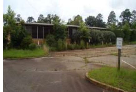
Peach Regional Hospital closed in 2013. Building was not salvageable. RDF funds demolished building; construction of hotel/conference center underway.
