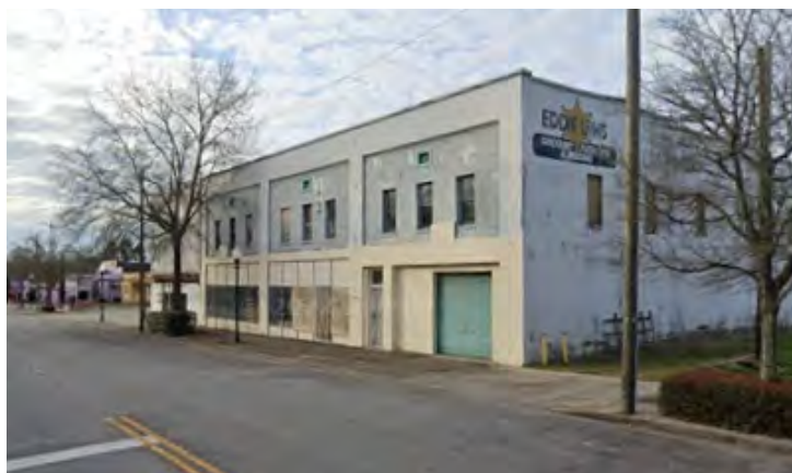
408 SOUTH PATTERSON STREET (CREDIT: GOOGLE STREET VIEW)
