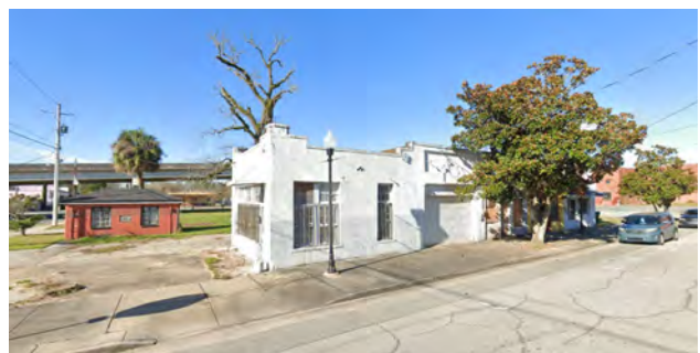
IMAGE: 422 SOUTH ASHLEY STREET (CREDIT: GOOGLE STREET VIEW)
