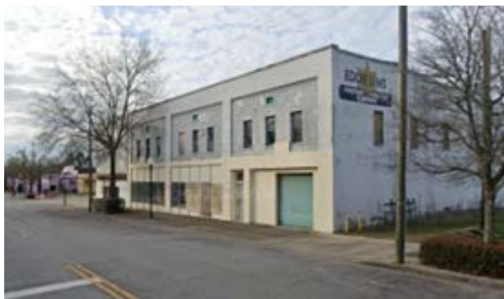
408 SOUTH PATTERSON STREET (CREDIT: GOOGLE STREET VIEW)
