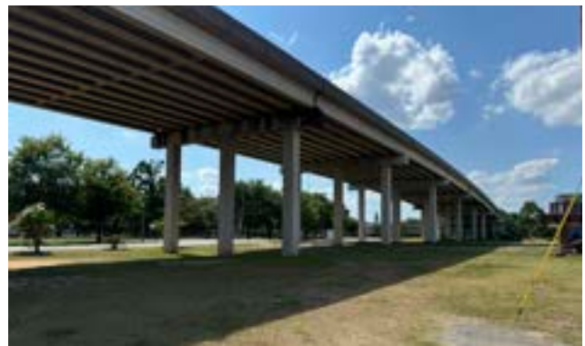
VIEW OF JIM BECK OVERPASS FROM OLYMPIC PARK
