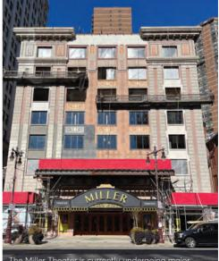
The Miller Theater is currently undergoing major renovations, including new windows. Notice the different colors of paint on the façade, used to help determine the building's new color scheme.
