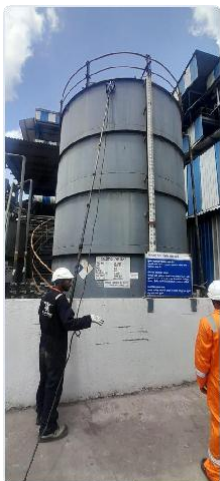
Figure 1: Ground-based UTM inspection of a tank shell using Reach Master, without scaffolding.
