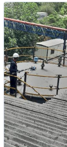
Figure 2: Remote inspection of a chemical tank roof, eliminating the risk of roof-collapse incidents.
