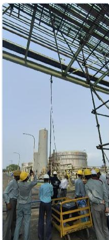
Figure 3: Team inspecting a high-altitude pipe rack using Reach Master
