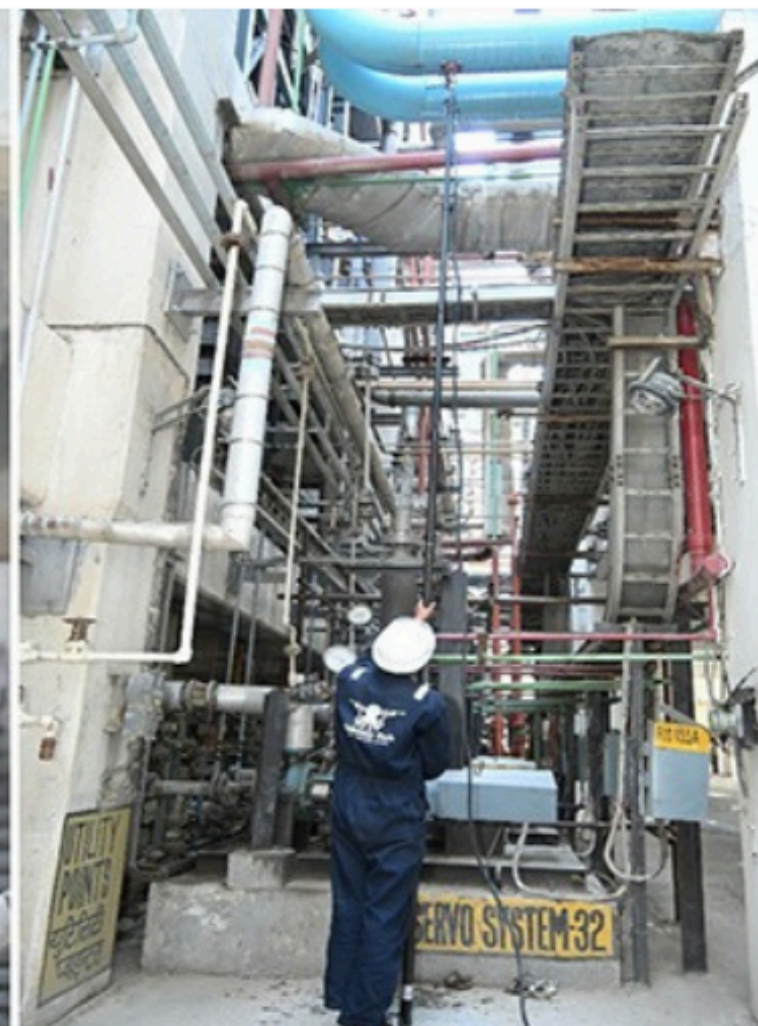
The system being used onsite (R)
