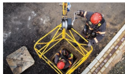
Vp plc ESS Safety, Survey, Test & Measurement
