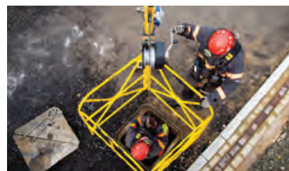
Vp plc ESS Safety, Survey, Test & Measurement
